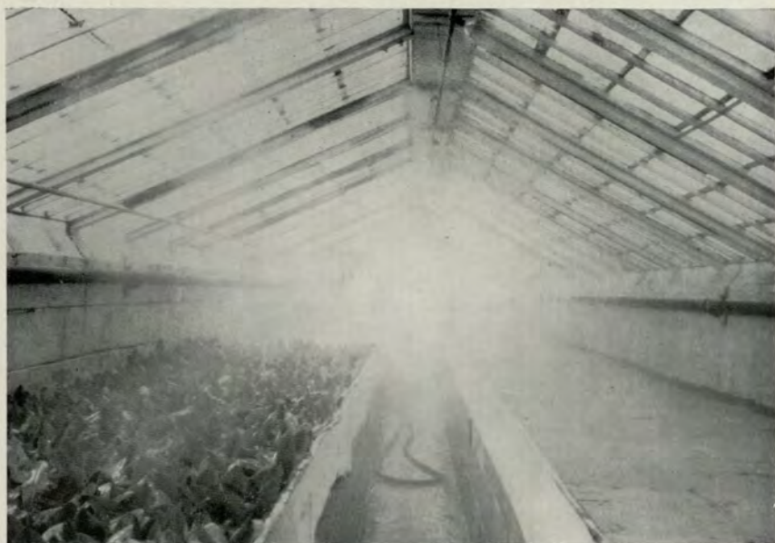
FIG. 29.—Humidification. The fog line is suspended below the centre board of the house. Jets are spaced 2 ft. apart and are directed alternately to either side. When in operation each jet needs 1\frac{1}{2} gallons of water per hour at 60-70 lb. per sq. in. pressure. Rhododendrons can be seen in position on the benches ( see p. 80 )
